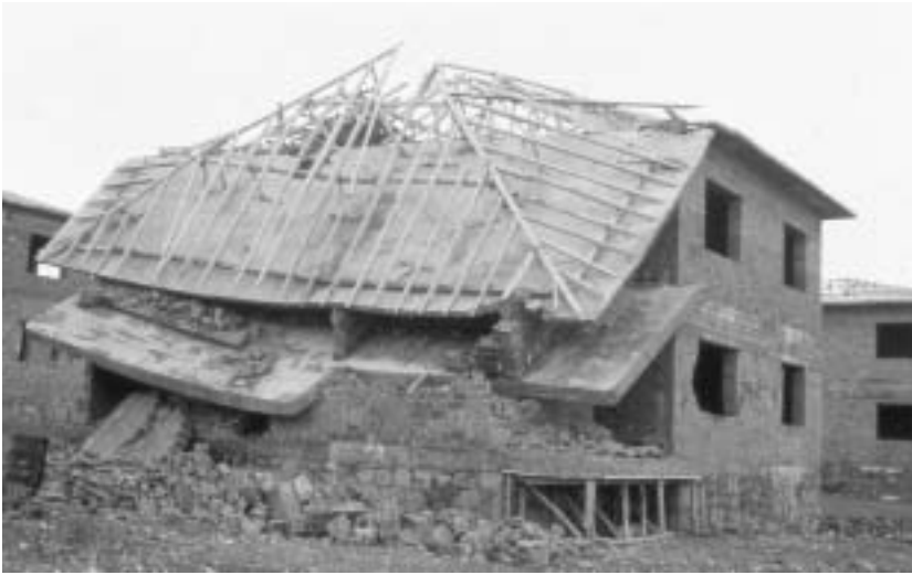
Fig. 10.2 Poor performance of hollow clay tile masonry in Erzincan, Turkey, 1992
