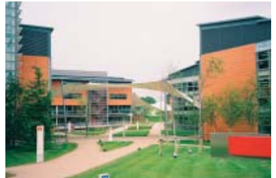
Fig 2.1 Vodafone's UK headquarters in Newbury provides a legible environment for easy orientation
